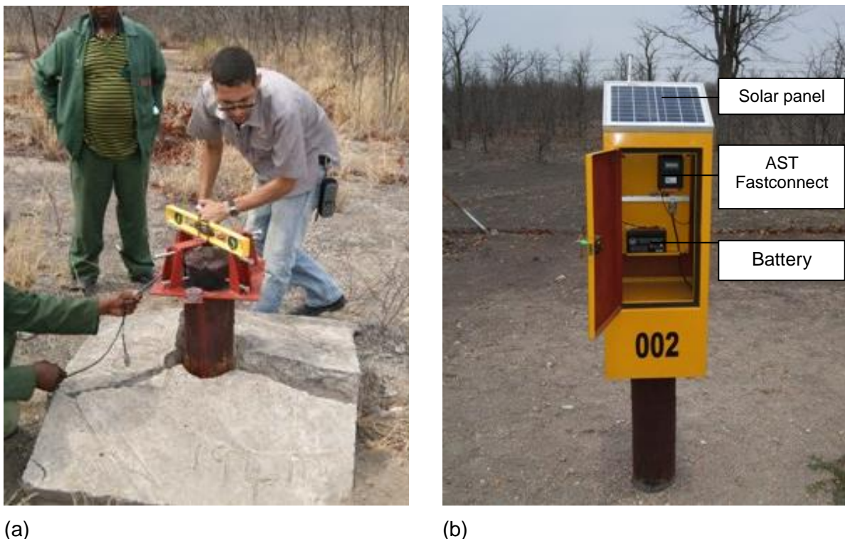
Figure 2 (a) attaching square base bracket to borehole casing (b) completed installation
