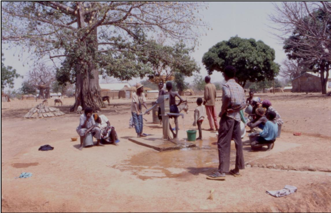
**Figure 2** A typical borehole in the Bolgatanga area fitted with an Afridev handpump.
