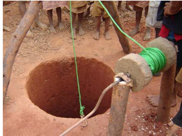
Well being dug through latasol weathered material
