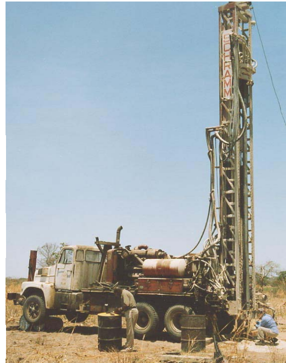
Borehole being drilled with down the hole hammer drilling rig
