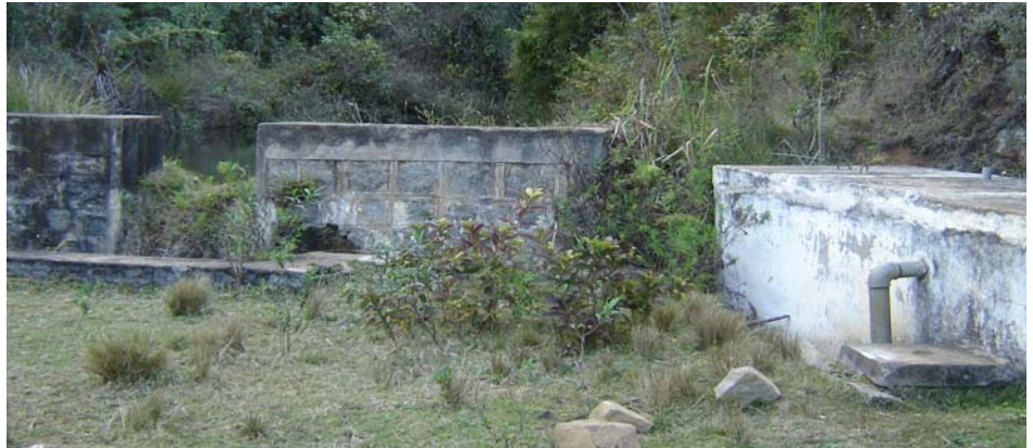
Spring outflow collection system with reservoir and outflow pipe
